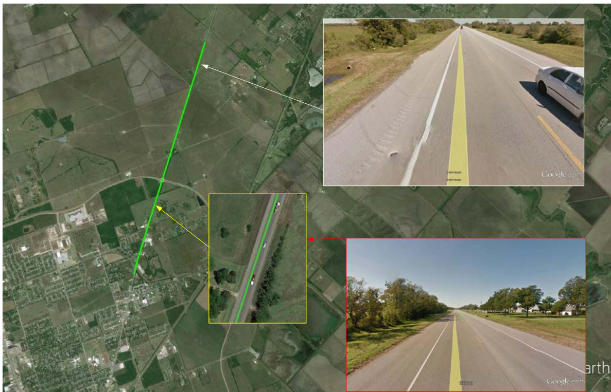
Figure 4. Segment in Houston District with Varying Shoulder Condition.
